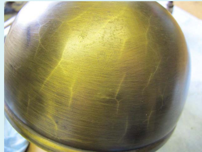
Image: A classic pattern of stress fractures on a boiler
